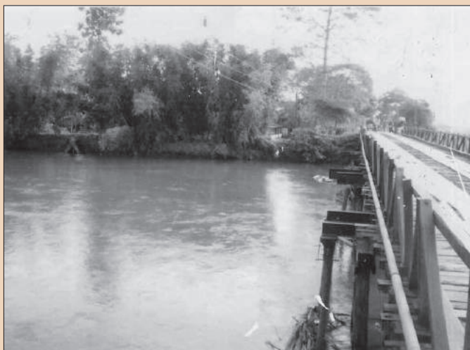
Figure 3. Bamboo planted along the river protects a major bridge.
