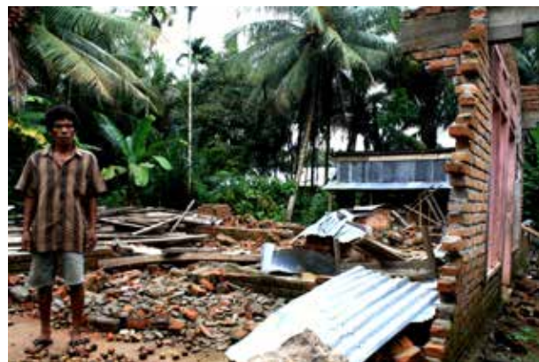
Destroyed home after earthquake in West Sumatra, Indonesia, 2009, Photo Credit: CRS
