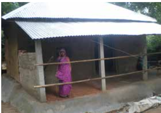
Completed flood-resistant shelter. Photo by CRS
