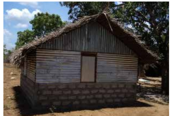
Completed transitional shelter Photo Credit: CRST
