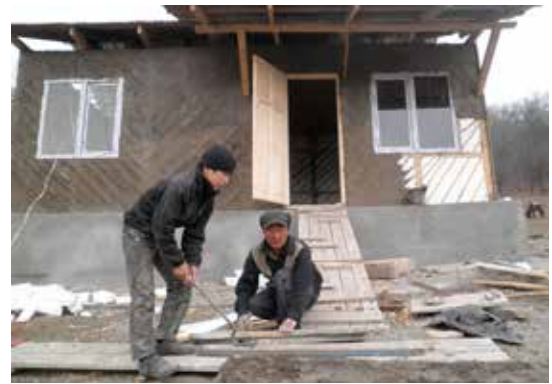
Winterized t-shelter with insulation layer under construction Photo Credit: Andrew Schaefer for CRS
