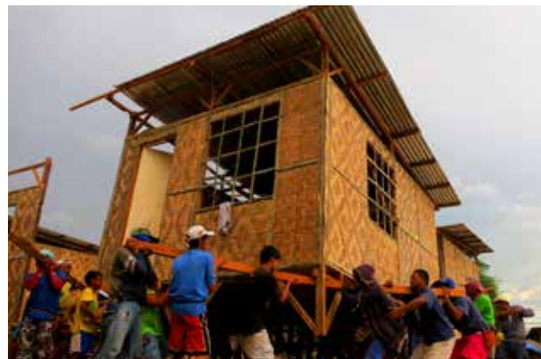
In Philippines shelter response, the transitional shelter was designed to be re-locatable and demountable Photo Credit: Charisse Mae Q. Borja for CRS
