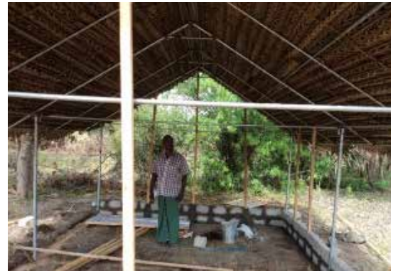
Construction transitional shelter Photo Credit: CRS
