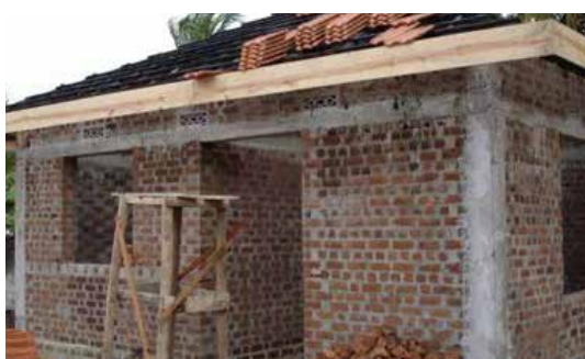
Permanent shelter in construction Photo Credit: Mehul Savla for CRS
