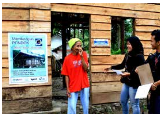
CRS team monitors the progress of T-shelter construction in Padang, west Sumatra, earthquake response Photo Credit: CRS
