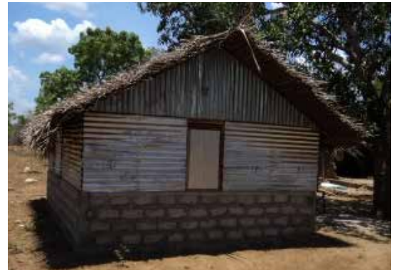
Completed transitional shelter Photo Credit: CRST
