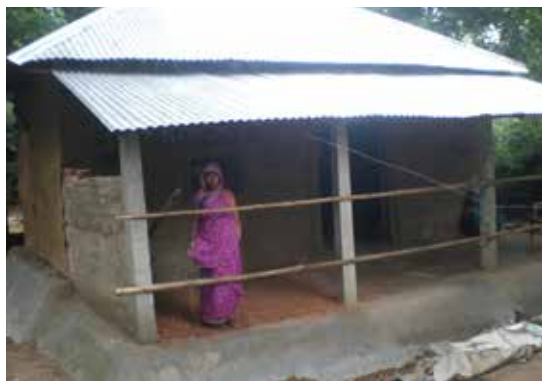
Completed flood-resistant shelter. Photo by CRS
