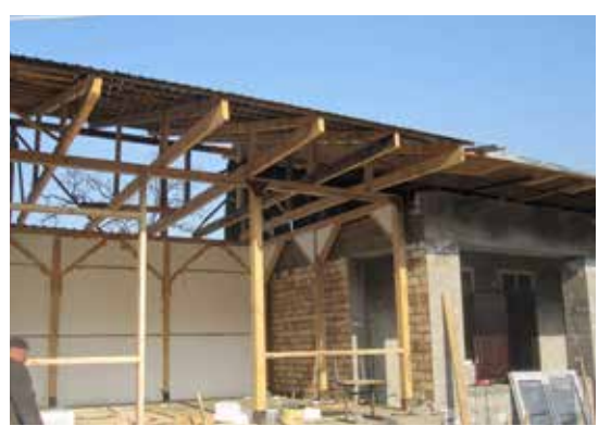
Winterized extensions to existing structures Photo Credit: Andrew Schaefer for CRS
