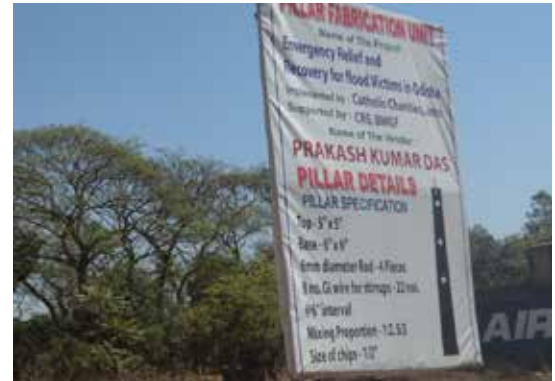
Reinforced concrete pillar prefabrication site for the structural frame of flood resistant shelter. Photo Credit: CRS
