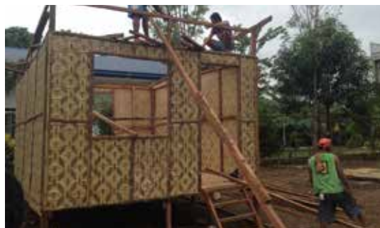
Pilot construction of transitional shelter Photo Credit: Andrew Schaefer for CRS
