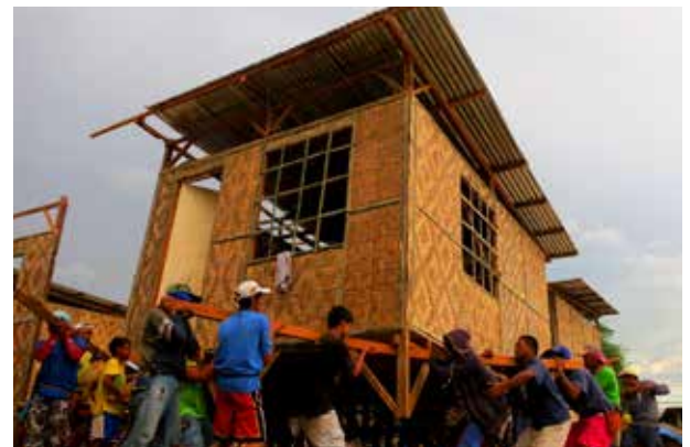
In Philippines shelter response, the transitional shelter was designed to be re-locatable and demountable Photo Credit: Charisse Mae Q. Borja for CRS
