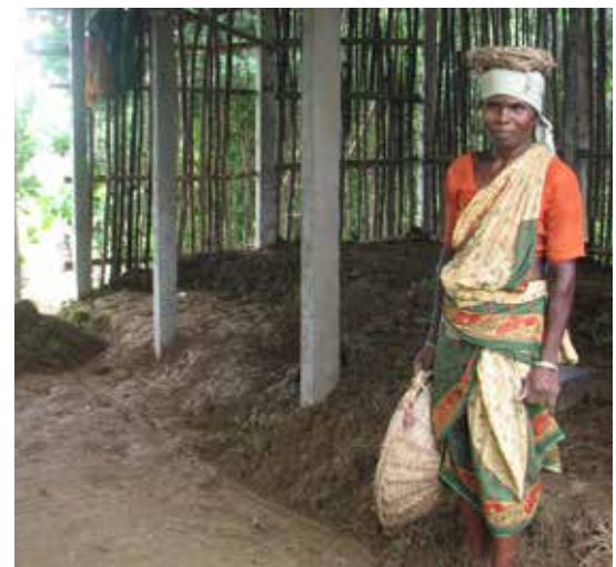
Owner creating the raised plinth around the concrete pillars. Photo Credit: CRS
