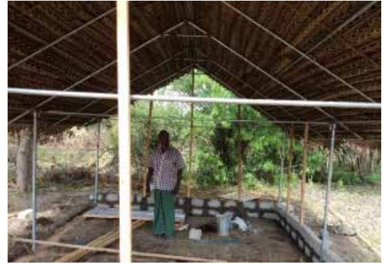
Construction transitional shelter Photo Credit: CRS
