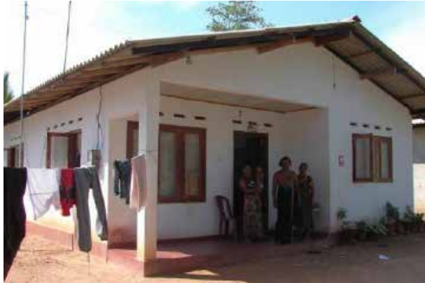
Pilot construction of transitional shelter in progress for post-tsunami shelter response, Sri Lanka Photo Credit: CRS
