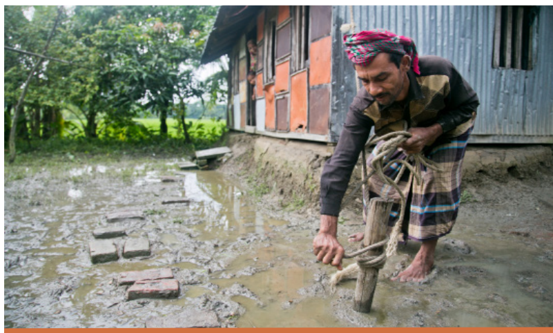
Almas Sikdar Almas secures his roof with rope, which will reduce flying debris in a storm. Jennifer Hardy/CRS
