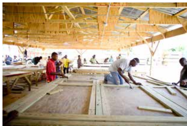
Local laborers built temporary shelter at Batimat factory, Haiti, 2010, Photo Credit: Benjamin Depp for CRS
