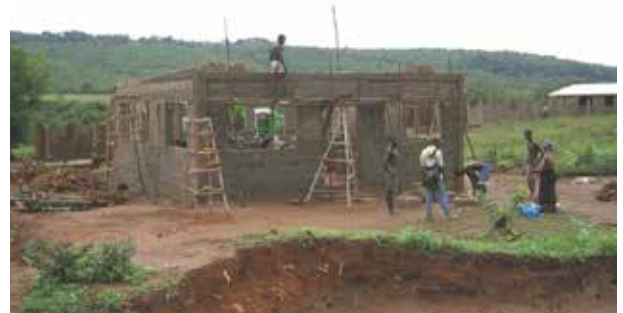
Permanent housing construction in progress in Sierra Leone, 2004 Photo Credit: CRS
