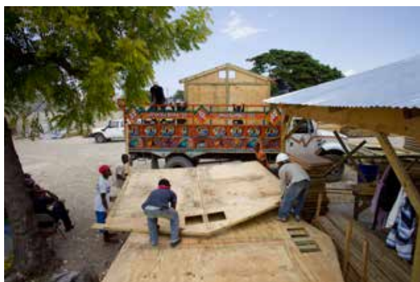
CRS partner Divine Ministries employees load a truck with sections of a transitional shelter at pre-fabrication yard in Batimal, Haiti, 2010, Photo Credit: Benjamin Depp for CRS
