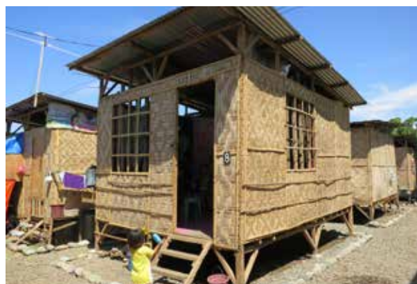
Transitional shelter in Philippines, Sendong Typhoon, 2012 Photo Credit: Andrew Schaefer for CRS
