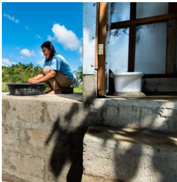
Left: The Type 6 toilet and septic tank is for households whose groundwater level is higher than 0.65 meters from the natural ground.
