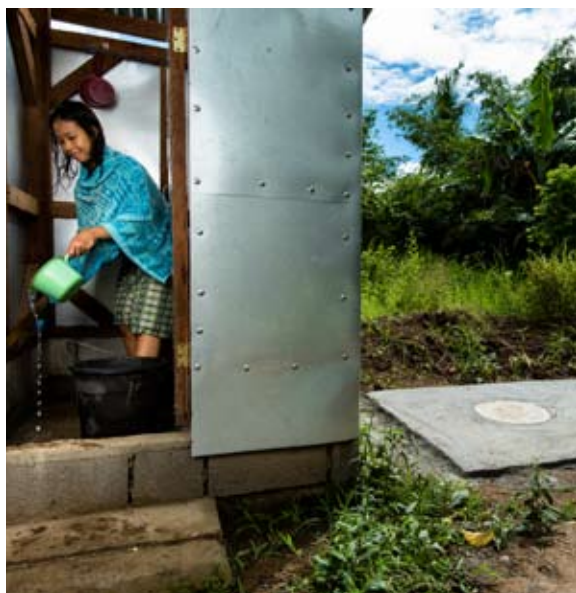
Above left: The Type 8 toilet and septic tank is for households whose groundwater level is below 1.5 meters from the natural ground. Above right: Anaerobic baffled reactors 5 were used for clusters of households where there was not enough space to build individual septic tanks.
