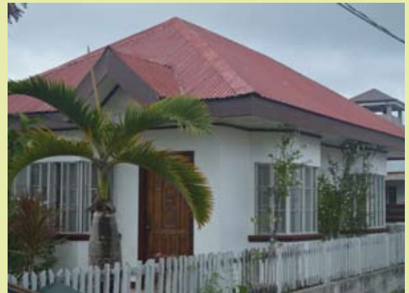
Households with “roofing only” damage received $423 to rebuild their homes.
