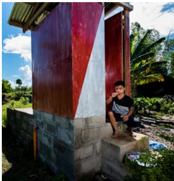
Below: The Type 7 toilet and septic tank is for households whose groundwater level is between 0.65 and 1.5 meters from the natural ground.
