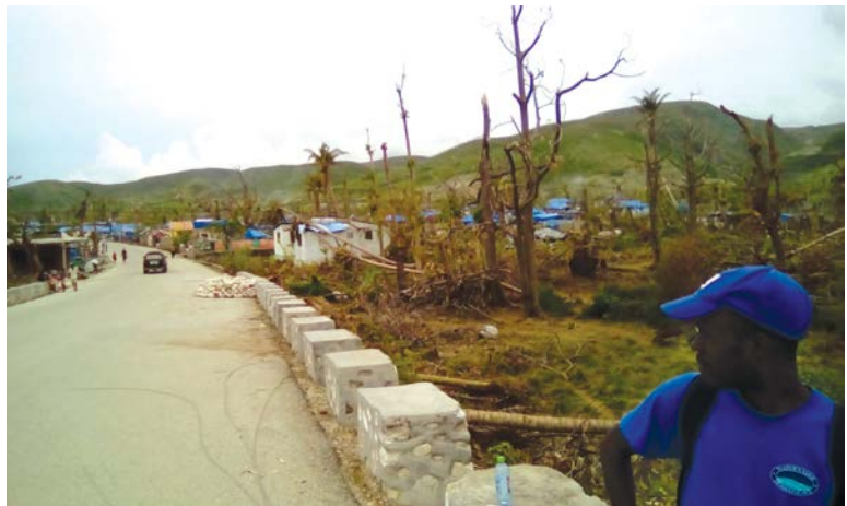
Tarp-covered houses, Damassin. CRS staff
